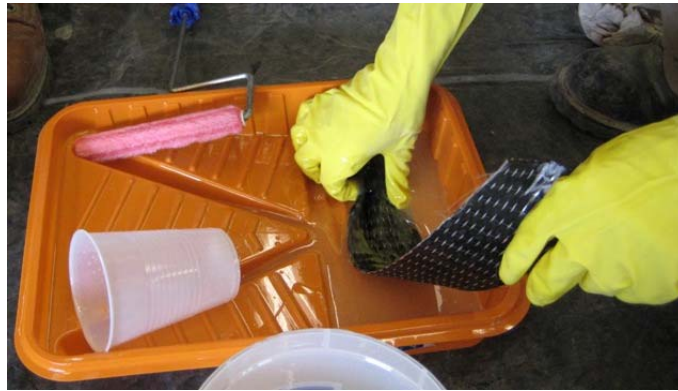
Figure 2.24 Saturating CFRP sheets
