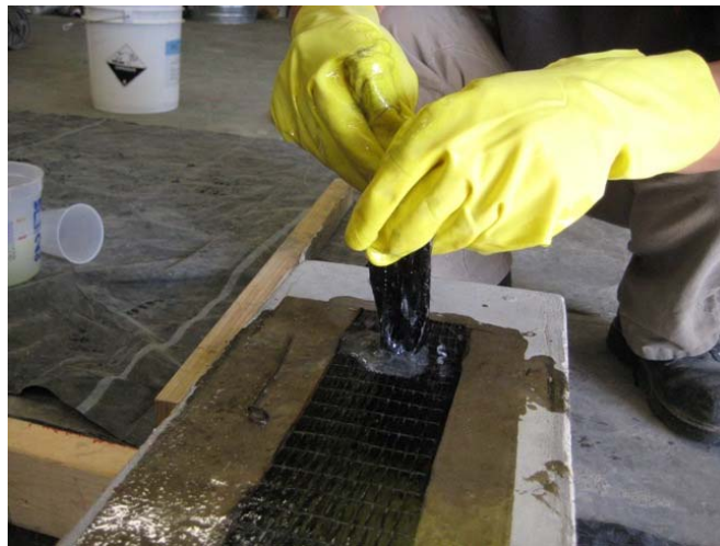
Figure 2.27 Inserting CFRP anchor into the hole
