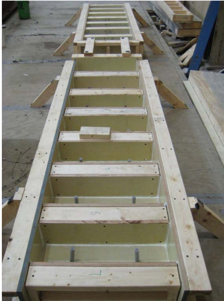
Figure D.1 Formwork for beam specimens
