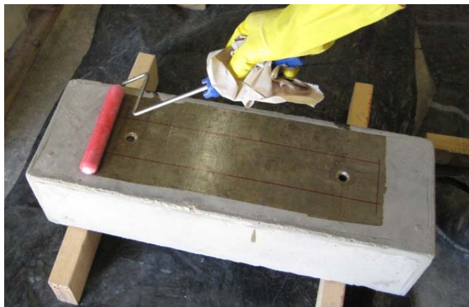
Figure 2.23 Saturating the concrete surface
