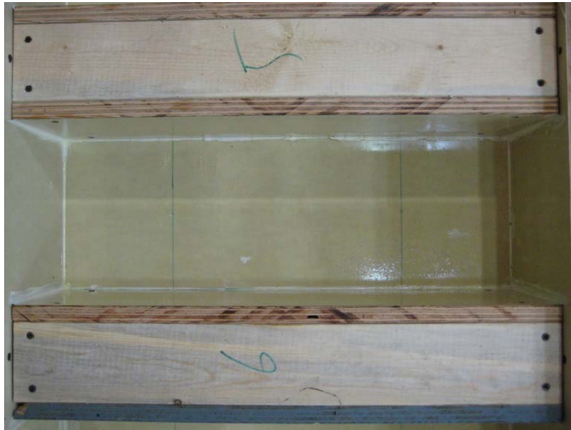
Figure D.2 Formwork
