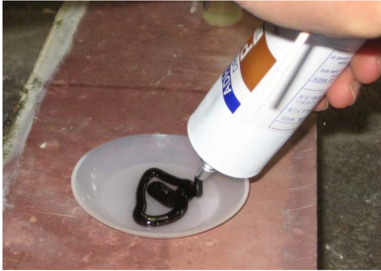
Figure B.2 Put Drug A of PS adhesive into a mixing vessel
