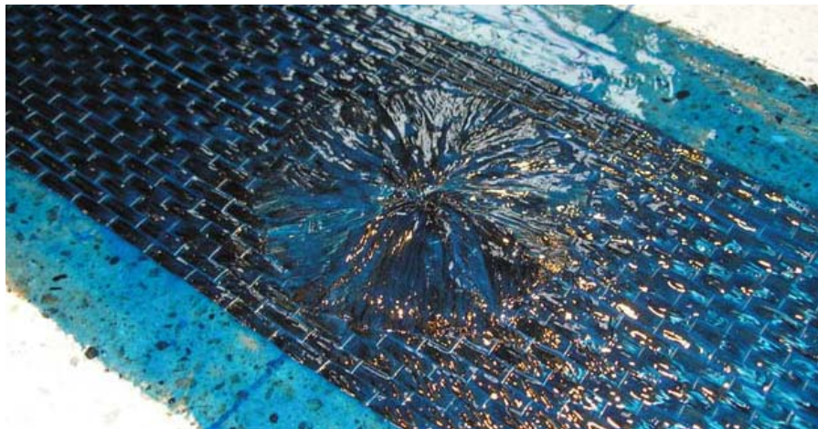
Figure 2.17 Use of 360-degree anchor fans [Niemitz, 2008 ]
