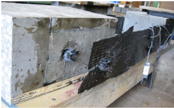
b) Fracture of CFRP anchor
