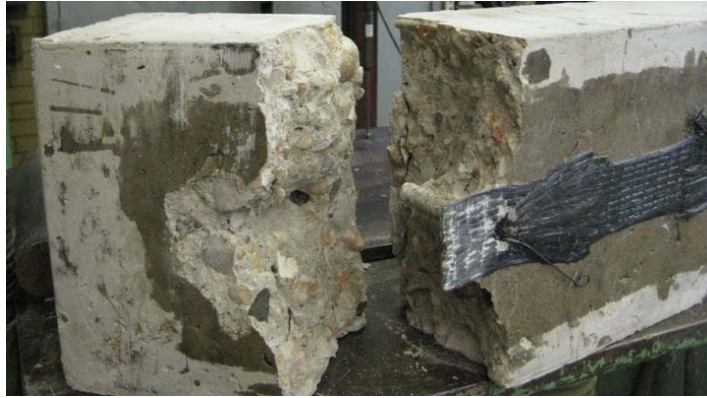
Figure 3.13 Detail of concrete failure
