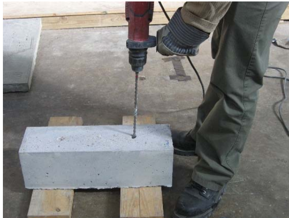
Figure 2.19 Drilling holes into the concrete element
