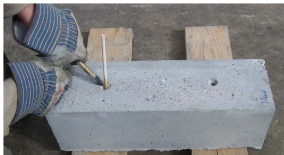
Figure 2.21 Cleaning the holes with compressed air
