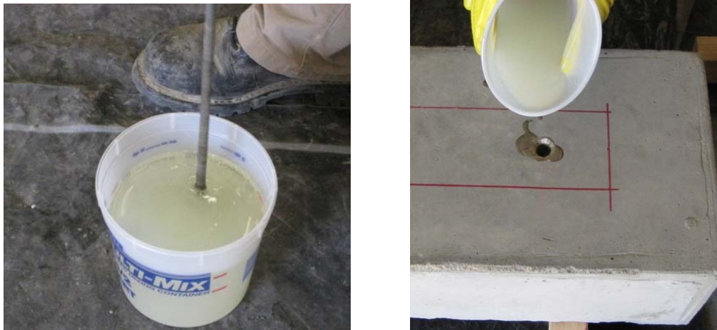
Figure 2.22 Mixing epoxy and saturating anchor holes
