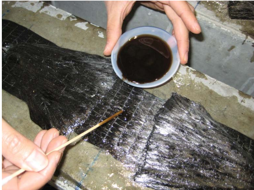
Figure B.4 Apply the mixed PS adhesive to CFRP laminate
