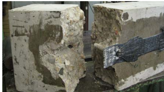
d) Failure of concrete behind the anchor
